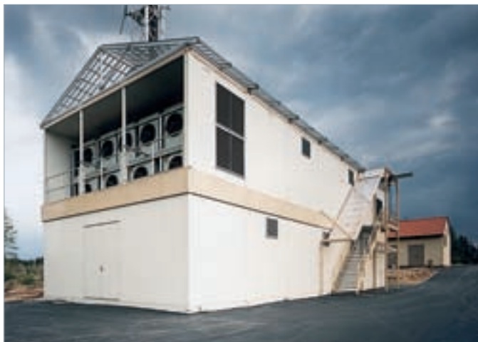
Main network transmitter station Remda/Saalfeld (Germany): two- storey transmitter building.
