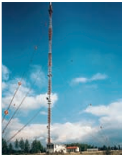
Overall view with transmitter mast.
