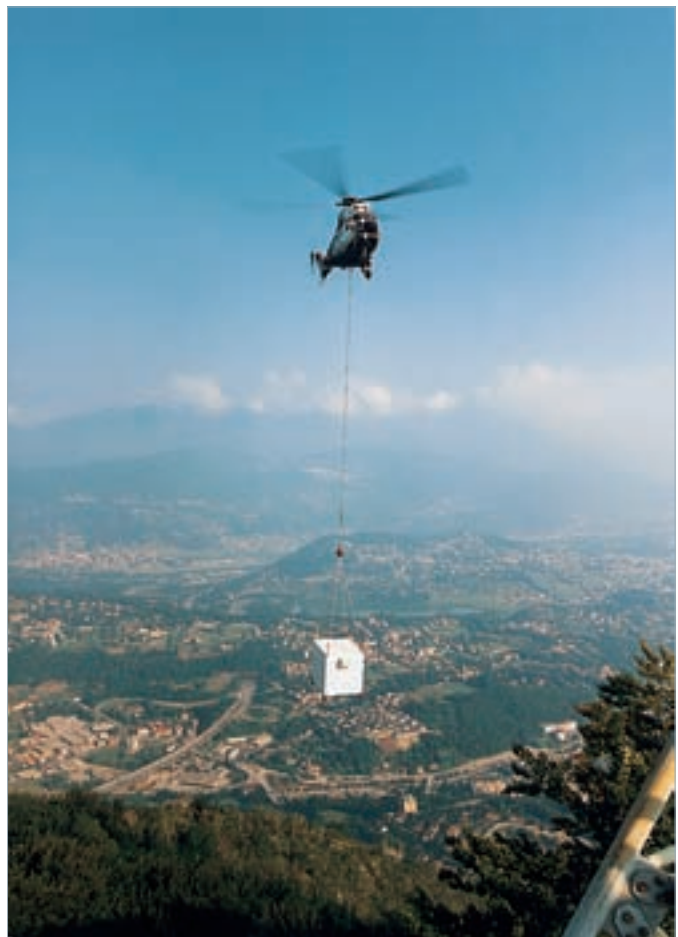
Transport of a 10 kW TV transmitter in container to San Salvatore station (Switzerland).
